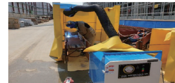
Installation of portable screen and dust collectors
